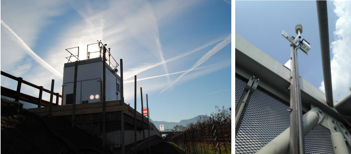
Figure 4 – Combination of conventional (left) and innovative low-cost (right) air quality monitoring stations in the BrennerLEC pilot test site.
